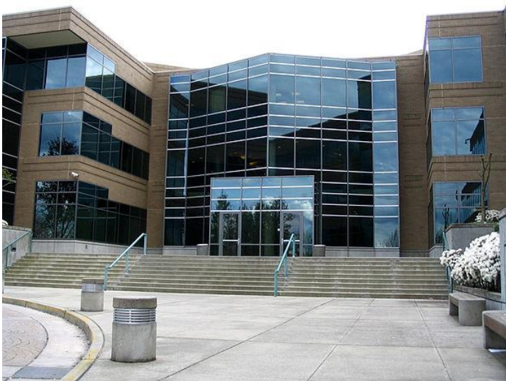
Lobby entrance of building 17
